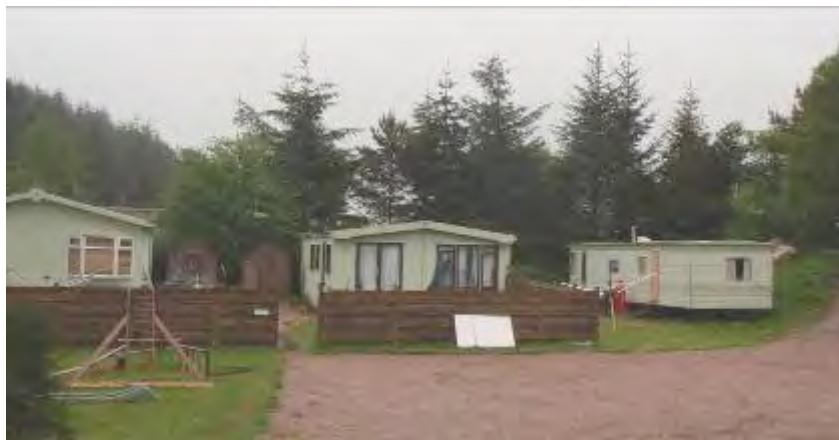
Fig. 2 : two chalet style static caravans, together with the caravan that is the subject of this current application (right)
